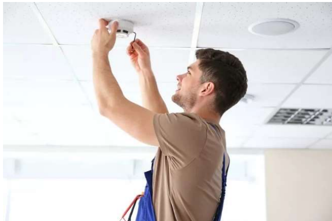
Slika 5: Montaža dimnih alarmov ( https://sl.your-best-home.net/7367041-smoke-detector-installation-what-costs-can-be-expected )
